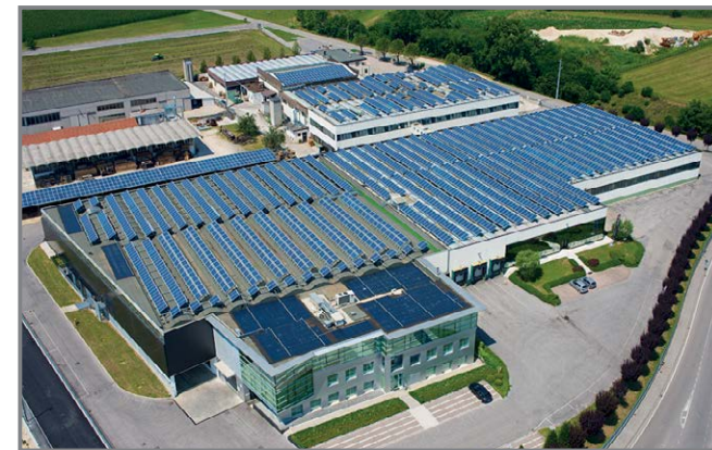
The roof the Grisport factory showing the extensive solar paneling
